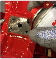
Clean the holes and the bolts (No1) with a degreaser solvent.
